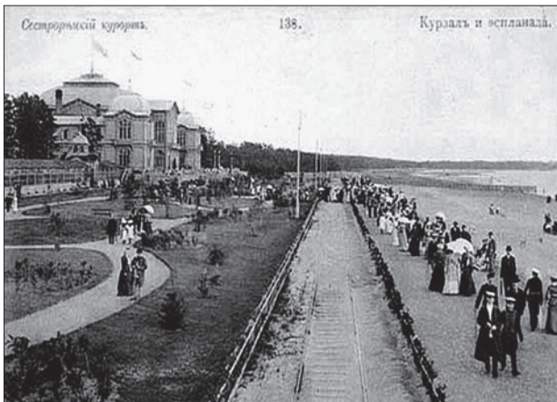
A part of the railway (St. Petersburg) was used as a line of electricity transmission
